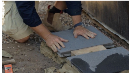
Place paver applying force to aid in bedding.
