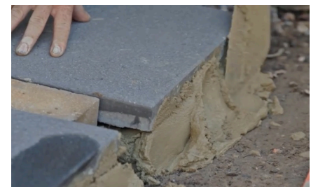
Haunching the sides of the pavers.
