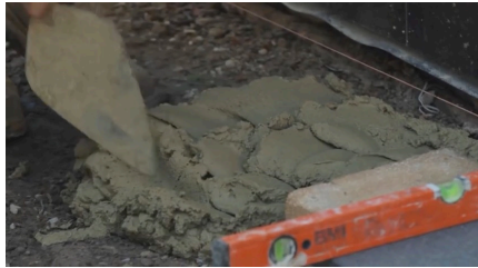
Spread thin layer of mortar for paver to bed on.
